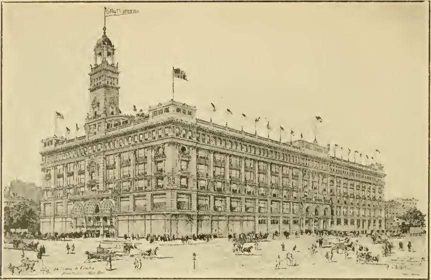
AN AMERICAN DEPARTMENT STORE. Exterior.
